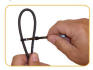
Create a loop on the uphole end of the cable and loosely bind it with one zip tie.
